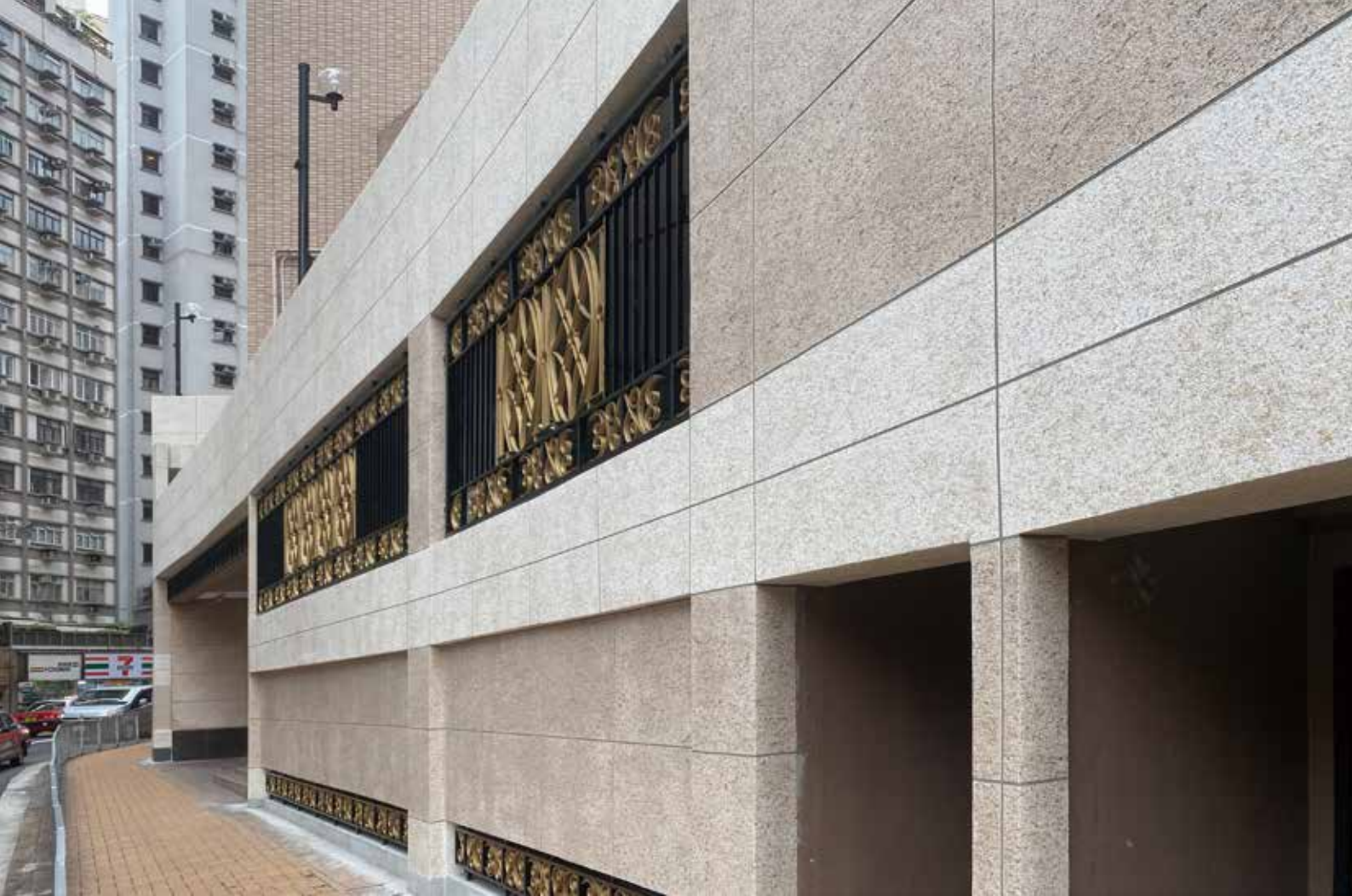
Ning Yeung Terrace, Hong Kong Finish: Shooting star finish m 2 : 1,500
